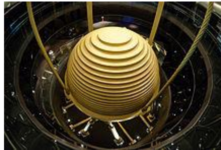
The main tuned mass damper atop Taipei 101
