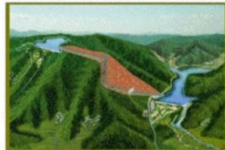
Pumped Storage Powerplant (Guaranteed capacity 50 MW)
