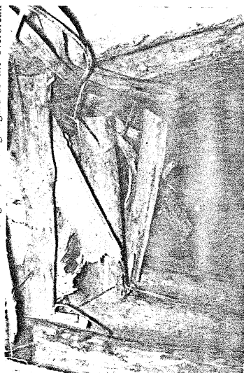
Fig. 17. Falling timber frames in the upper heading in the first tube of the Serra Ripoli super-highway twin tunnel, Italy
