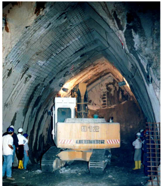
Fig. 20: Side drift in the Athens Metro Olympion station excavation.
