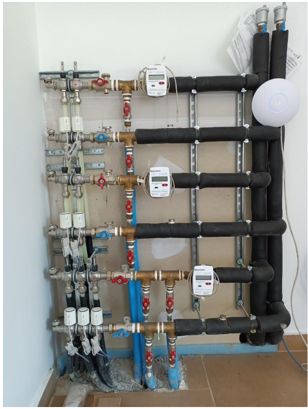
Distribution manifold (selection between underfloor and fan-coil units)
