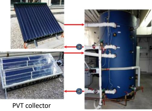
Rated power 10 kW Thermal efficiency COP=0.5 Adsorbent Zeolith Hot water inlet temperature from PVT 55oC Hot water inlet temperature from vacuum collectors 95oC
