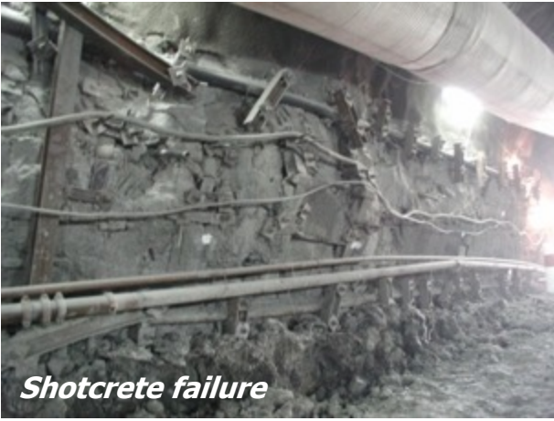
Steel set yielding due to the overstressed tunnel support section
