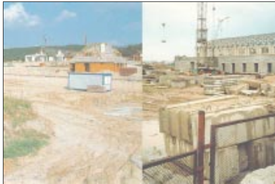
Fig. 26 Representative demonstration of the quoted class on examples of houses and technical objects under construction in Slovakia and Lithuania
