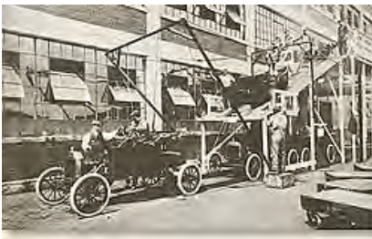
Assembly Lines for cars, 1913
