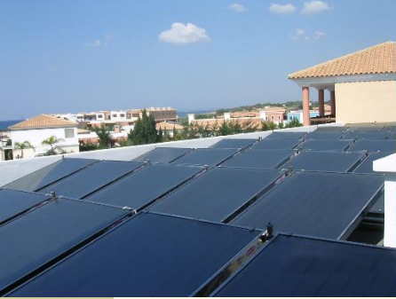
Solar system for domestic water heating and heating support (System: flow heater)
