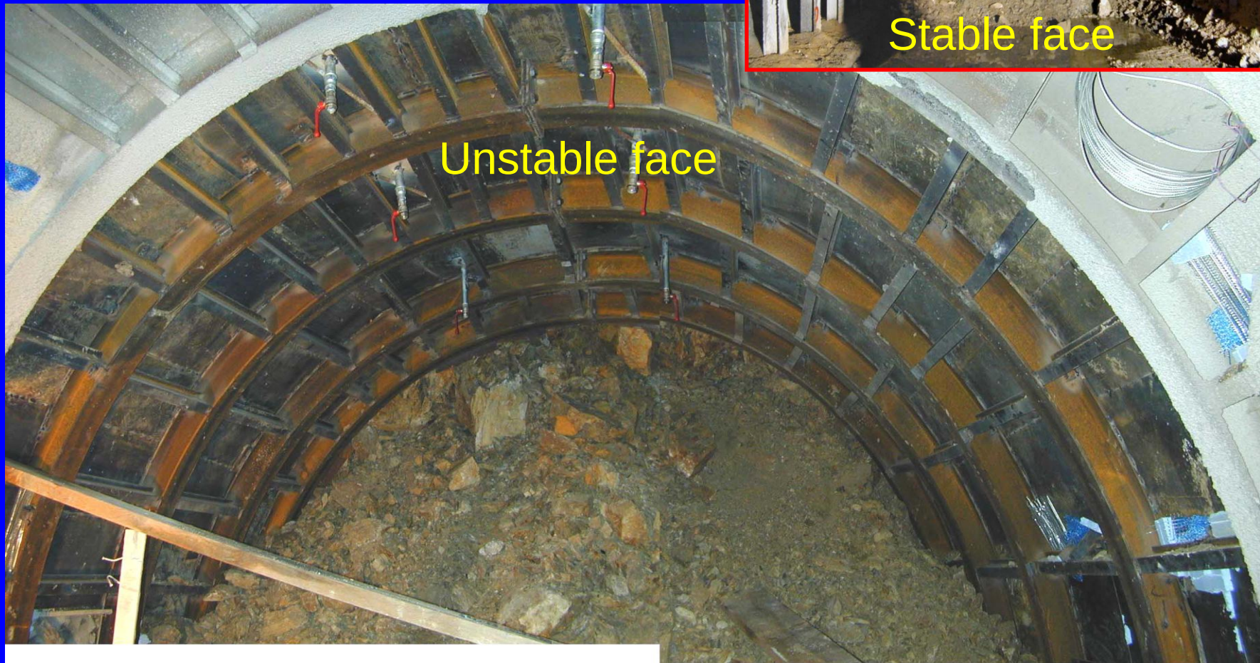
(1) Crown failure
