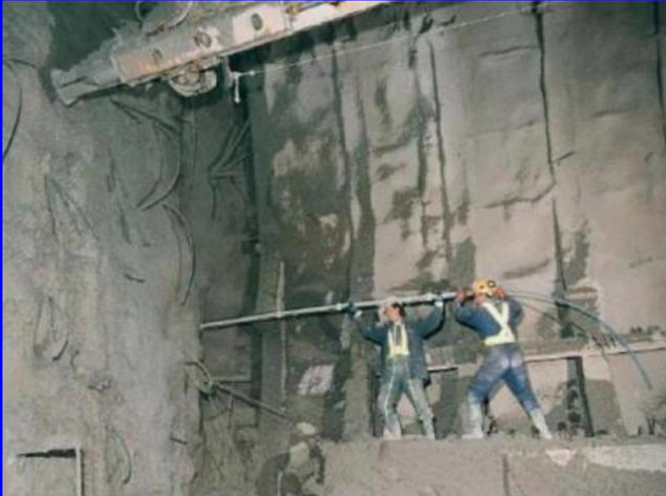
Installation of Fiber-Glass nails on tunnel face
