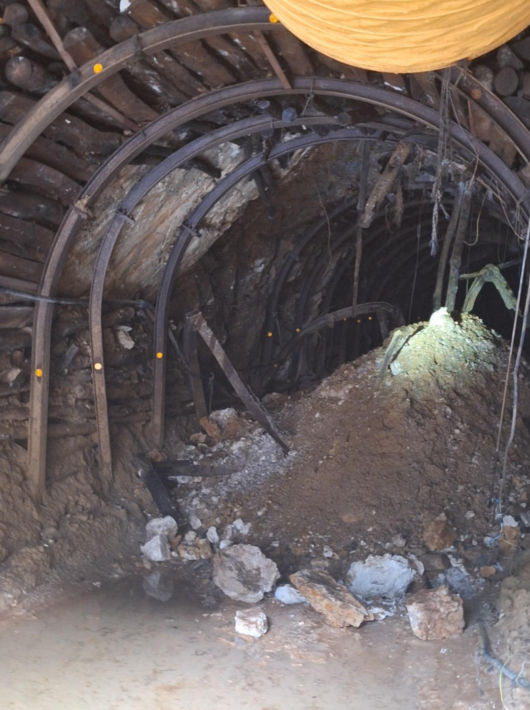
"Old" Austrian Tunneling Method
