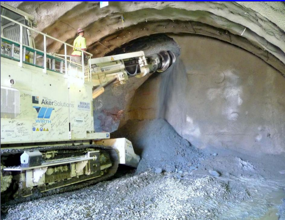
Mechanised tunnel excavation (TBM)
