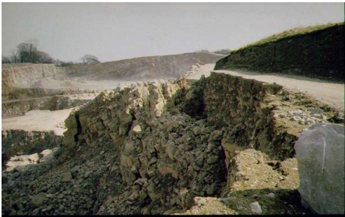
Figure 65. Example of an accident due to no adequate design of a road or poor monitoring
