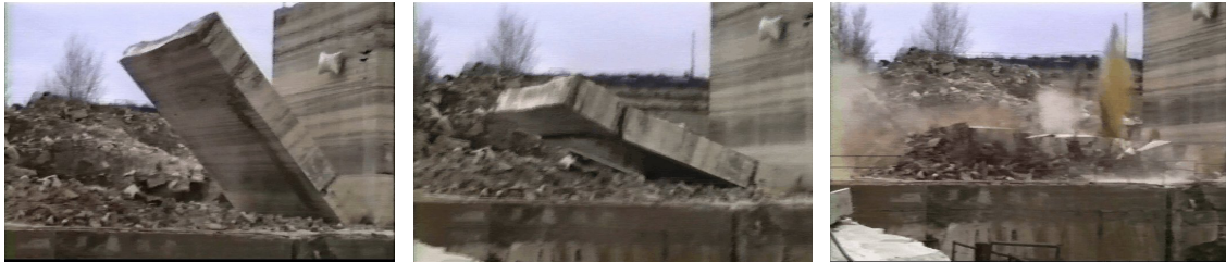
Figure 75. Overturning of a bench (courtesy of G. Saviano)
