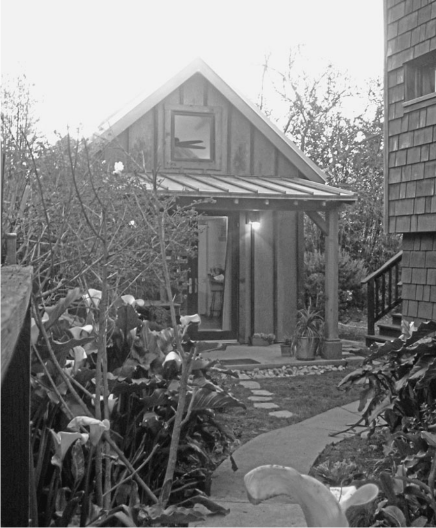
Figure 3.2 My backyard cottage, built under Berkeley's accessory dwelling unit law Photo credit: Karen Chapple
