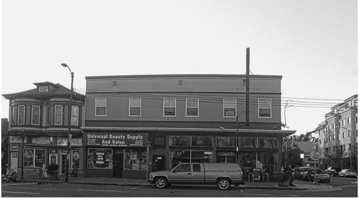
Figure 3.1 Infill development in Oakland, California
