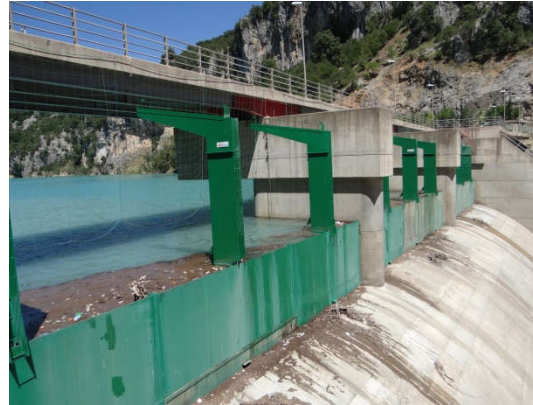
Spillway and fusegates
