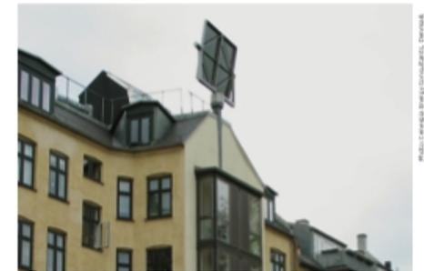
Novel use of a solar mirror to direct skylight down into the communal stairwell.
