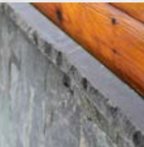
Figure 11: Align adjacent pieces of stone along a particular plane.
