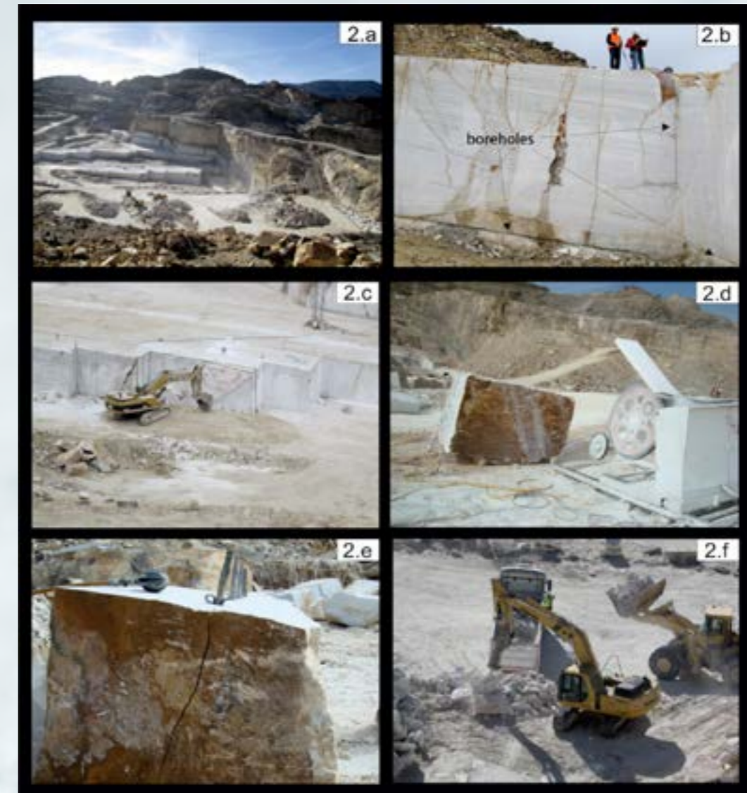
Figure 1.2. a) Overview of a quarry; (b) Details of the three perpendicular holes that delineate the secondary bank; (c) Cutting of tertiary blocks with a diamond wire (detail of the block is outlined). Excavator extracting blocks over the sand bed. Note the breakage along a fracture plane; (d) Squaring a block with a diamond wire; (e) Squaring a block with a drill and wedges along a crack; (f) Excavator with a hydraulic hammer reducing the size of the stone intended for micronized carbonate. (Martinez et al., 2017).
