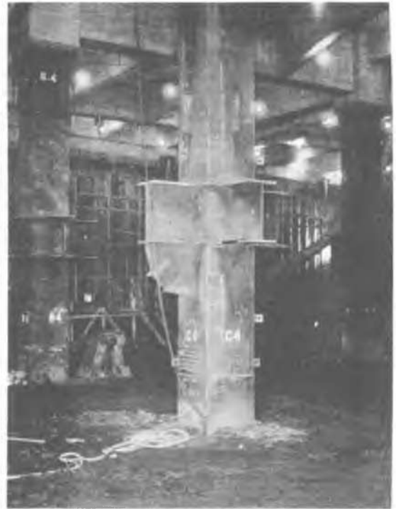
Fig. 18. Inside View of a Floating Island Method
