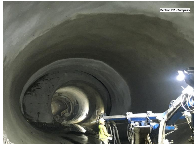
Figure 24 FRSC lining complete
