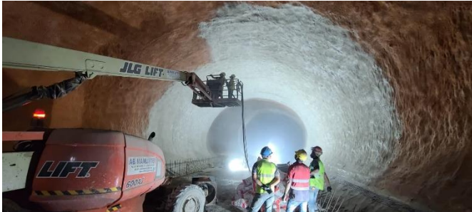
Figure 23 Sprayed waterproofing membrane 2 nd pass complete
