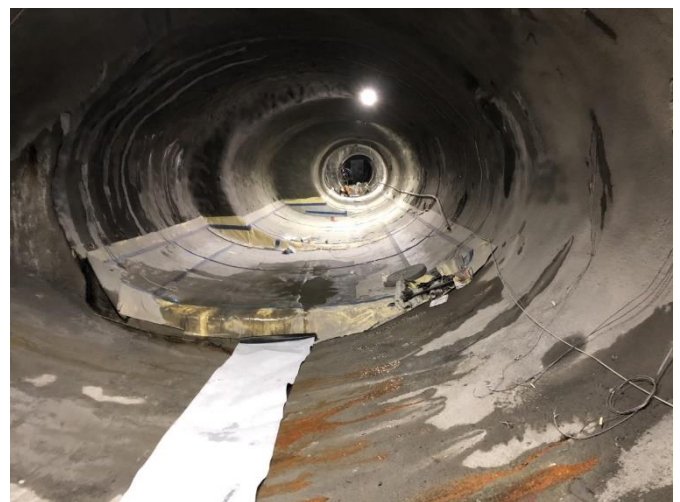
Figure 20 Invert temporary water management and drainage collection
