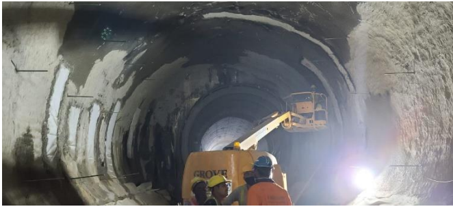
Figure 21 Installation of water management details prior to spraying
