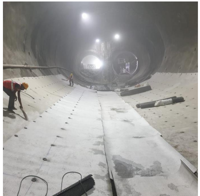
Figure 19 Invert under-membrane water management installation
