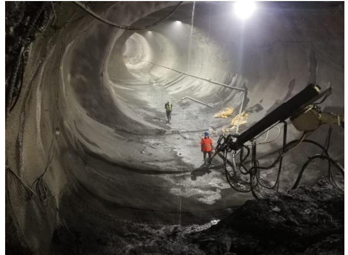
Figure 18 Primary lining complete. Invert drainage and temporary sump construction
