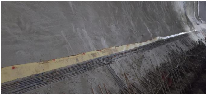
Figure 22 Invert/arch waterproofing termination construction
