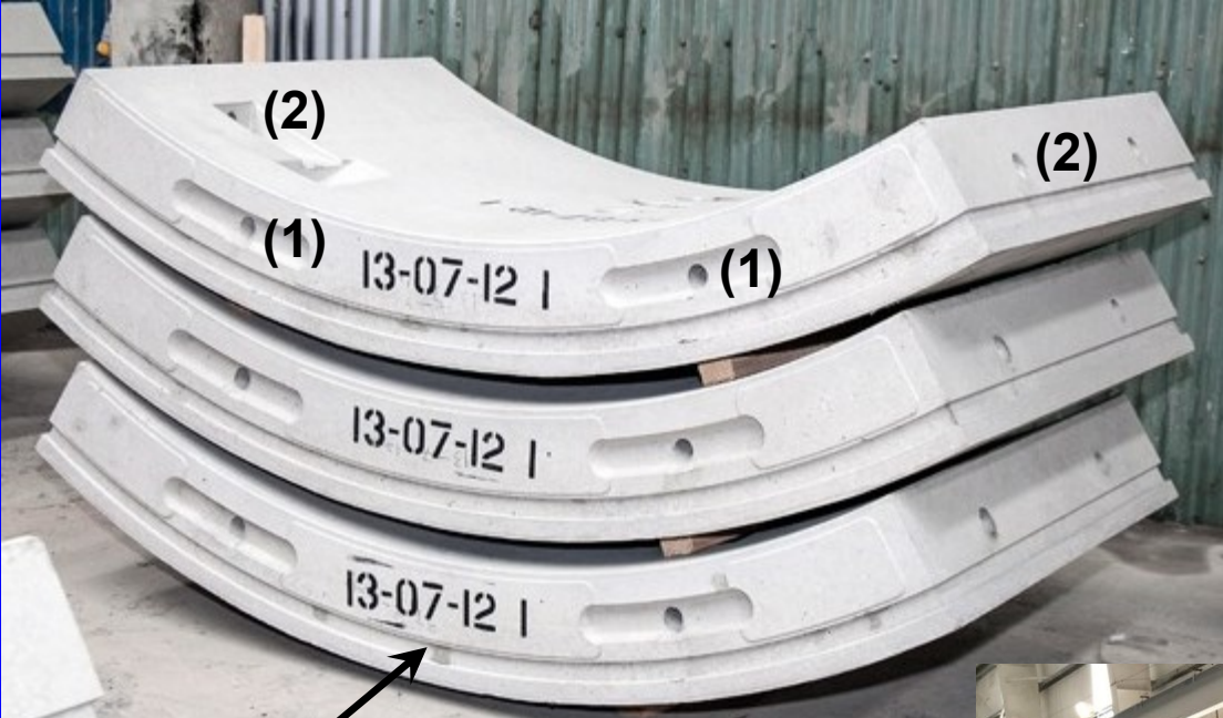
Groove for waterproofing gasket
