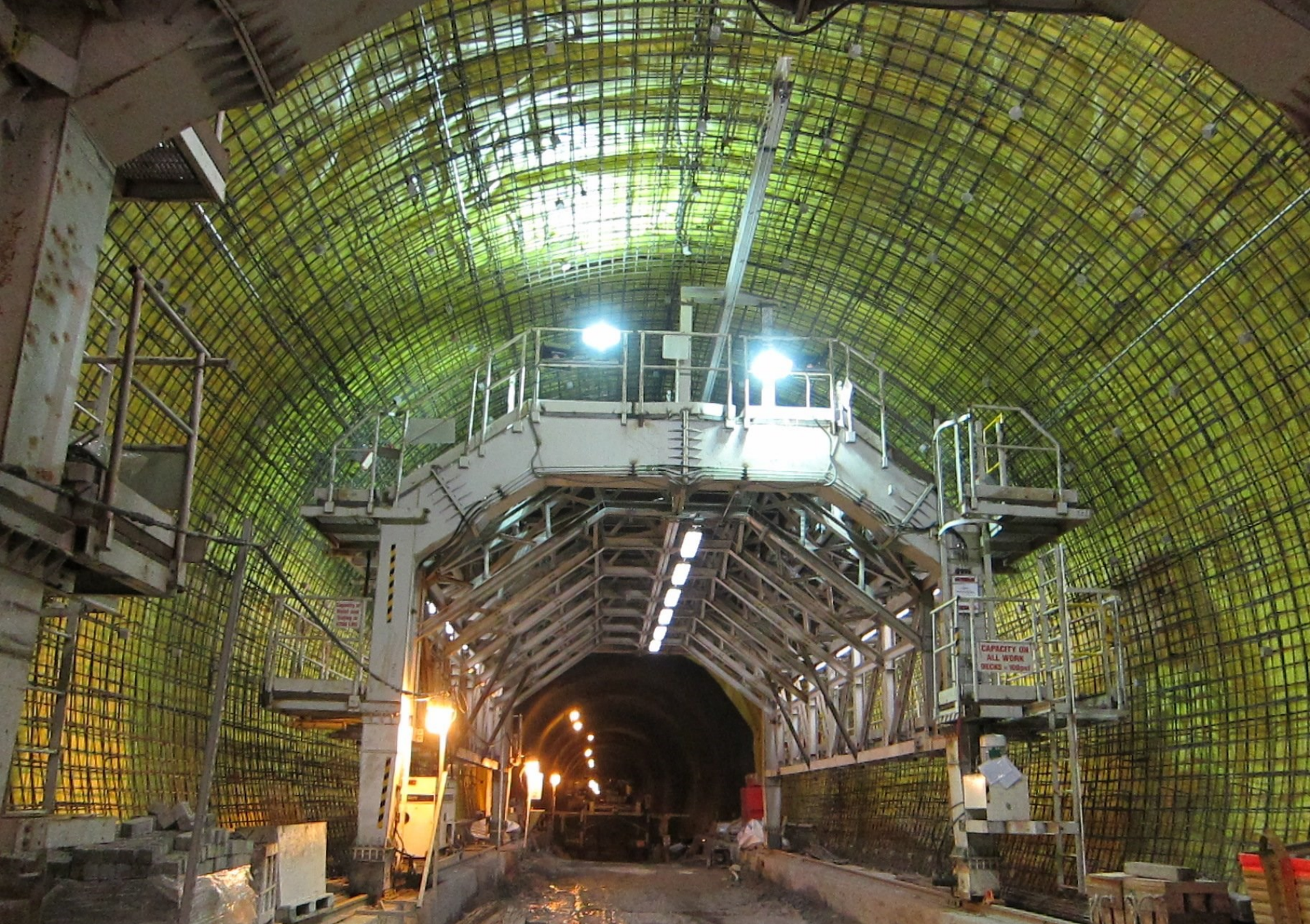
Final lining of tunnels – Erection of steel reinforcement
