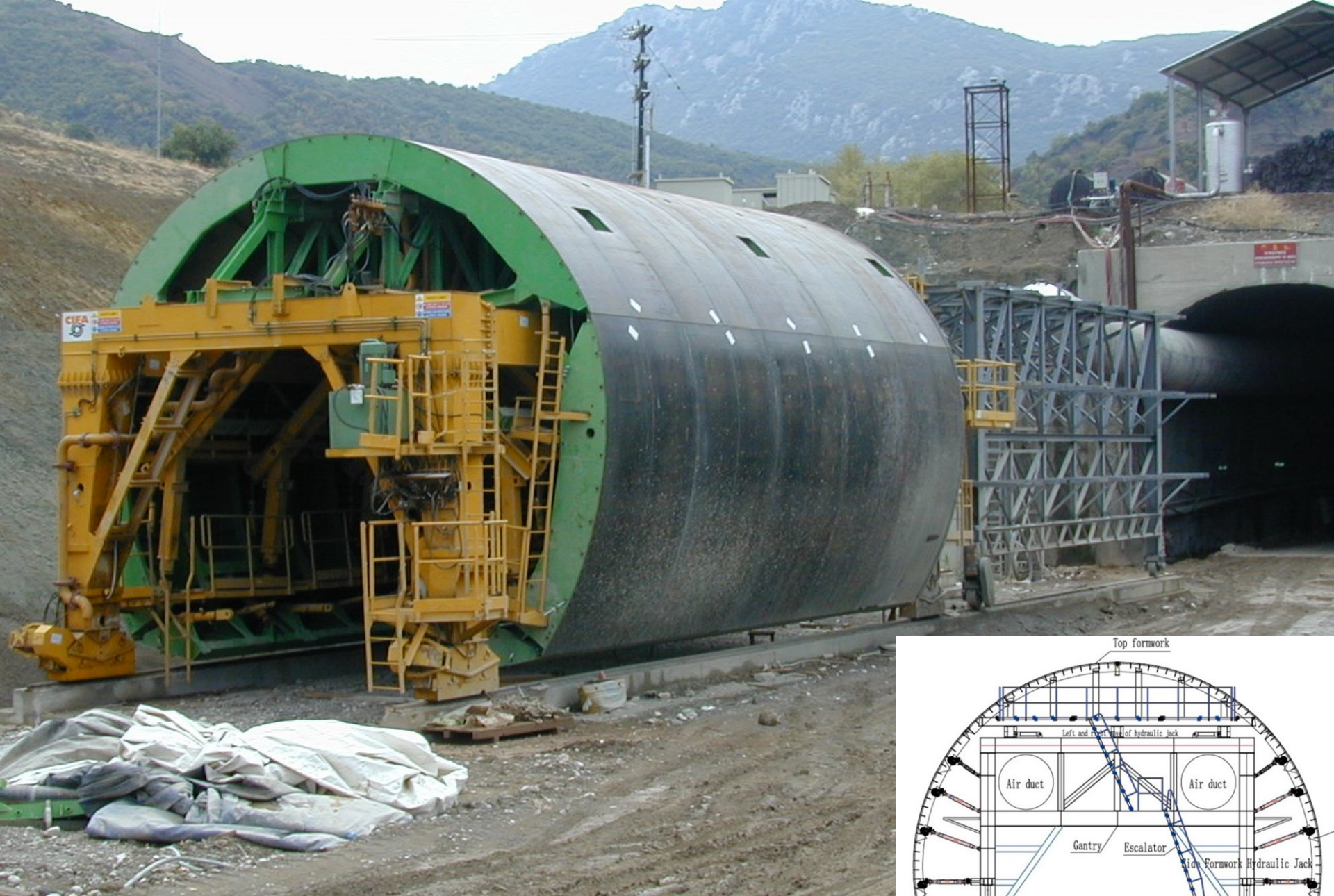
Final lining of tunnels – Rolling metal form for concreting and erection platform of steel reinforcement
