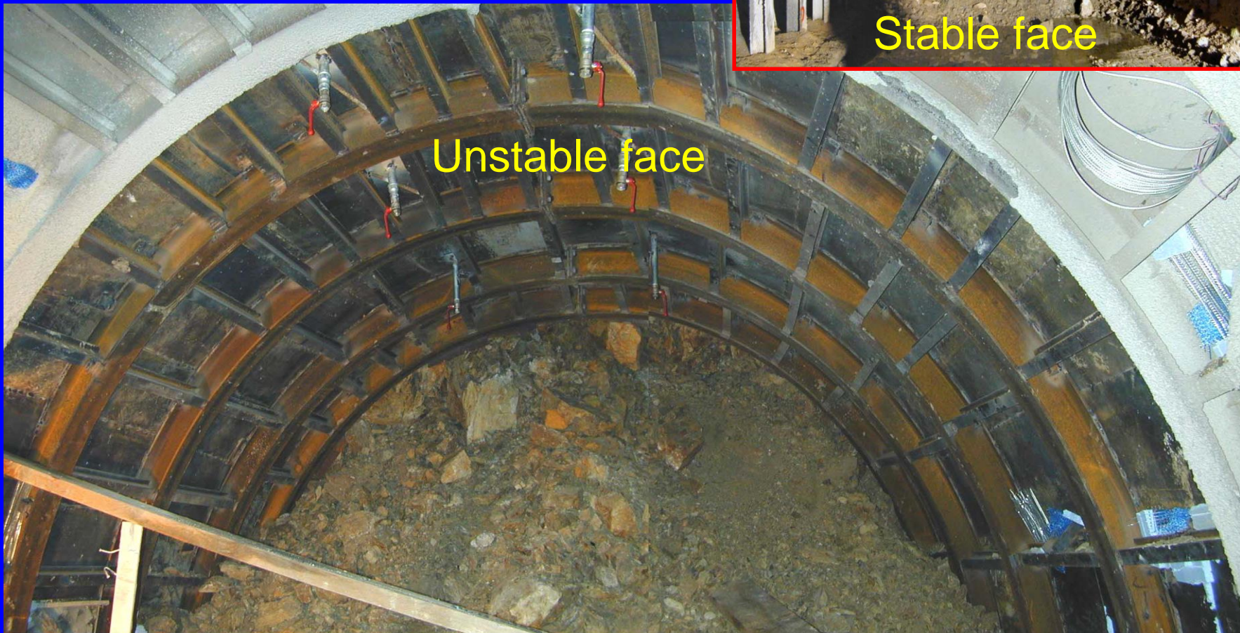
(1) Crown failure
