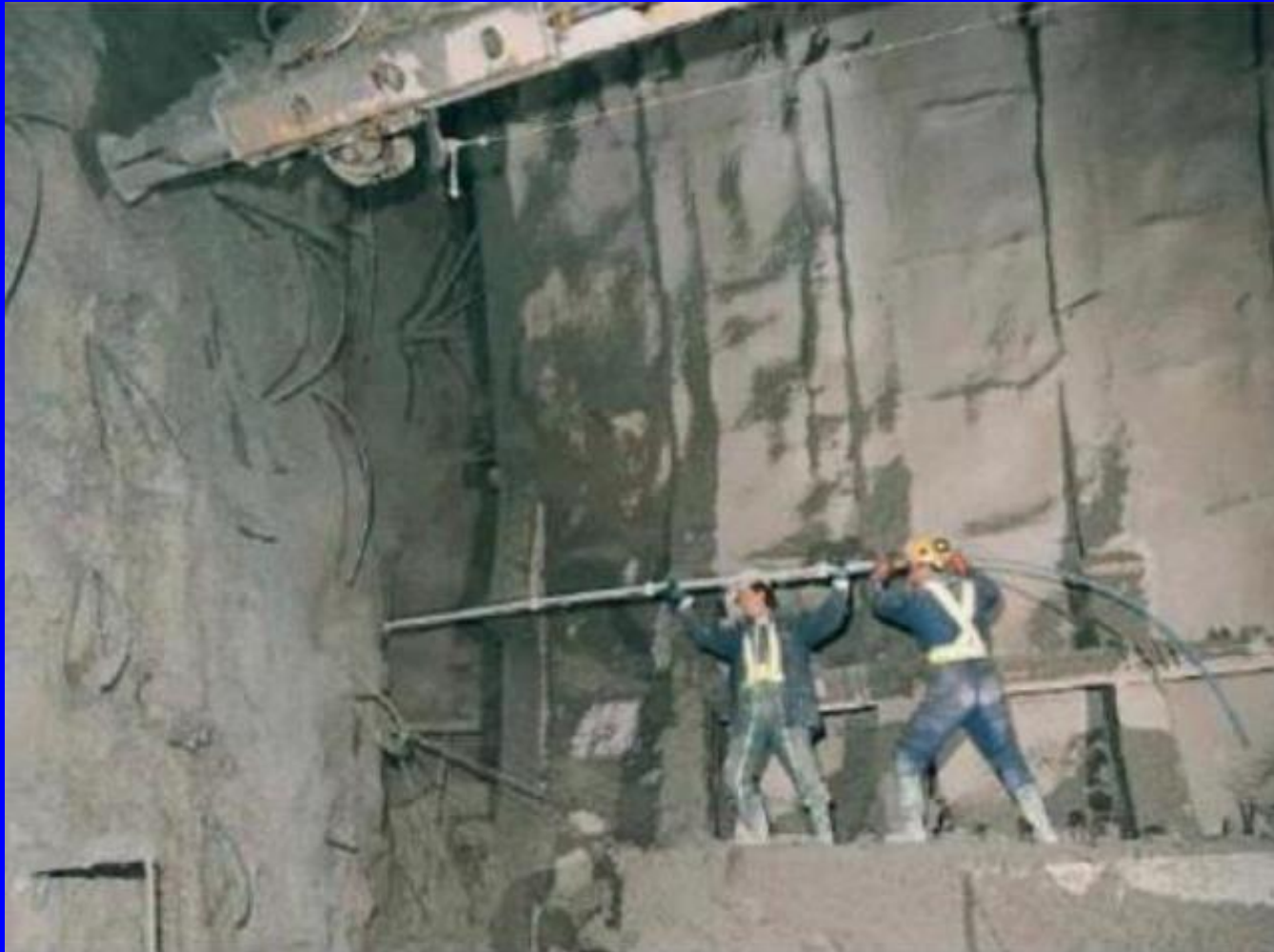
Installation of Fiber-Glass nails on tunnel face
