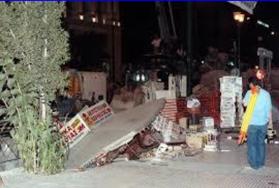
Athens Metro, Panepistimiou Av. Catastrophic TBM face collapse (1997)
