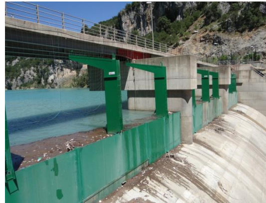
Spillway and fusegates
