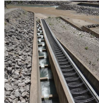
Fish ladder and small boats passage
