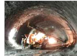
Driskos highway tunnel, Greece
