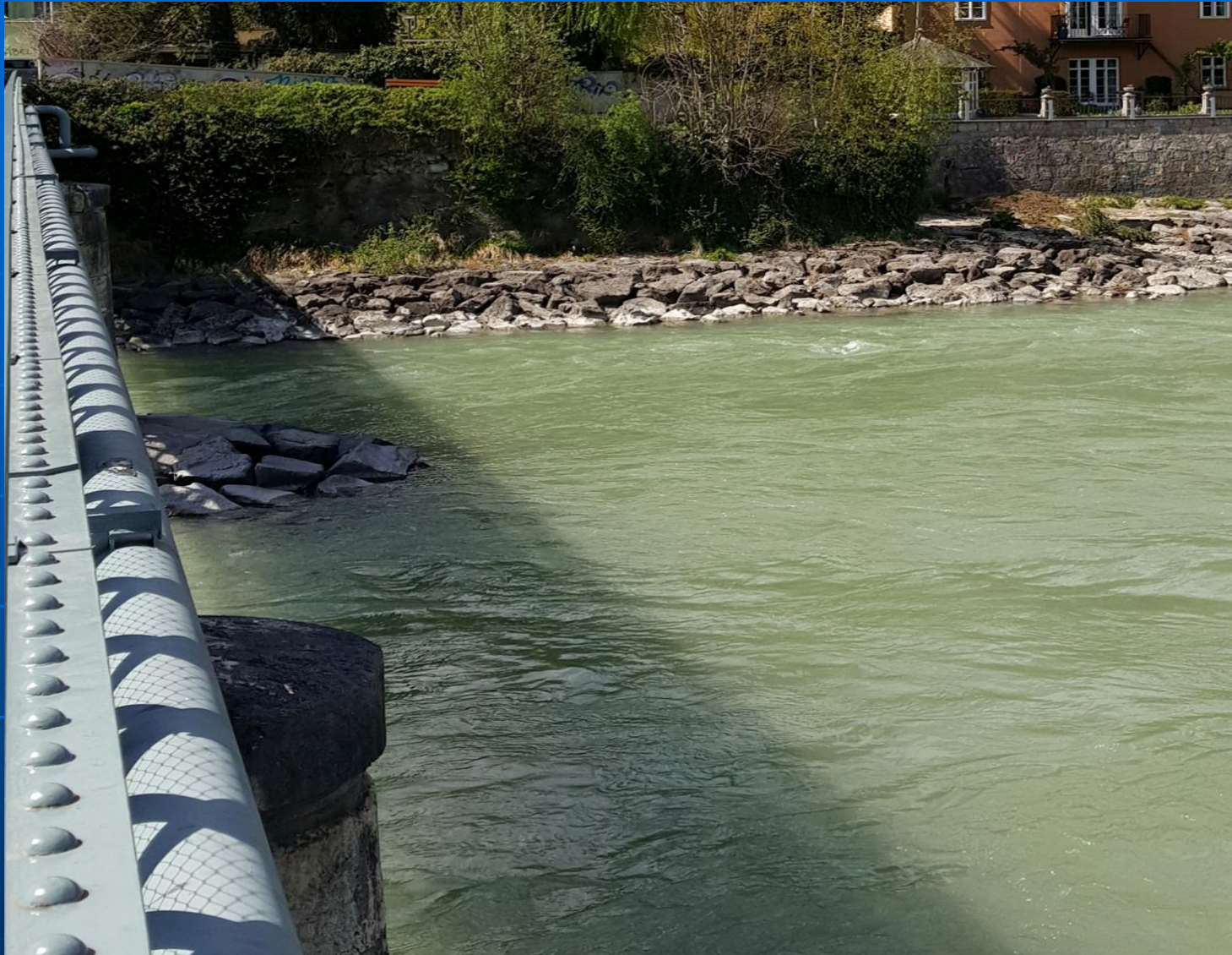
Pier protection of scouring
