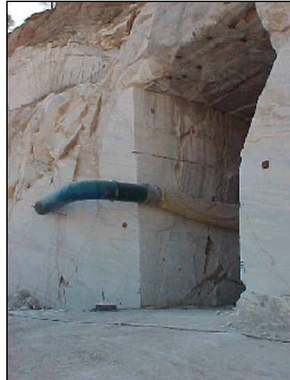
Figure 63. The intake (fan) of the ventilation system.
