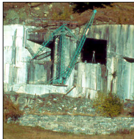
Figure 35. Opicalcite underground quarry (Italy).
