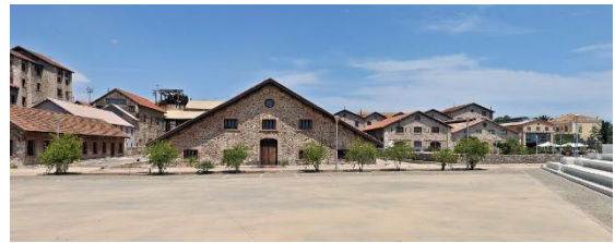
Figure 2. Lavrion Technological and Cultural Park (LTCP)
