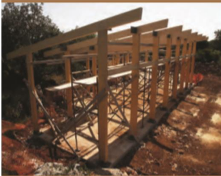
laminated timber structural frame
