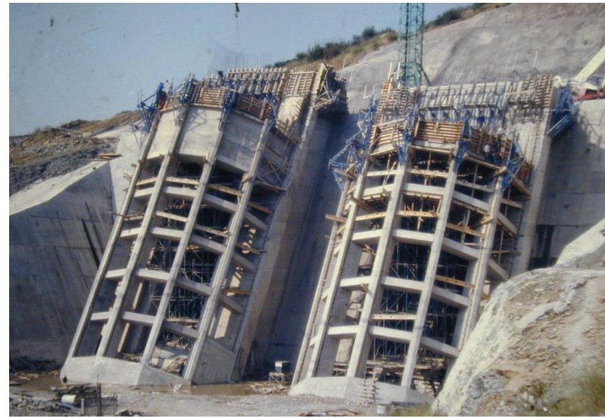
Stratos dam: inclined intakes under construction
