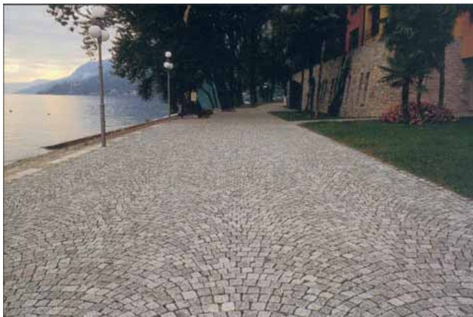
Figure 47. Example of granite sets use for external paving.
