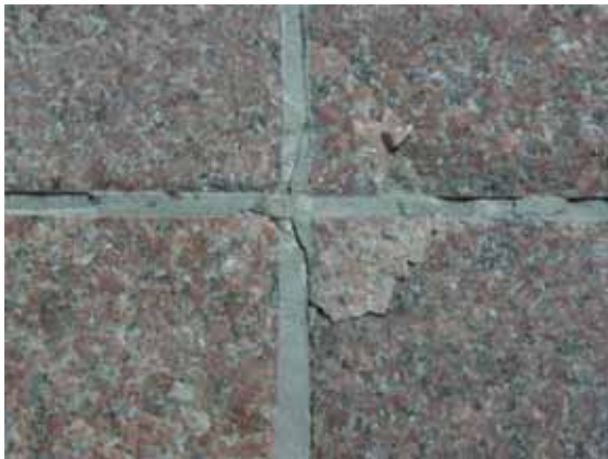
Figure 142. Damage caused by thermal dilatation
