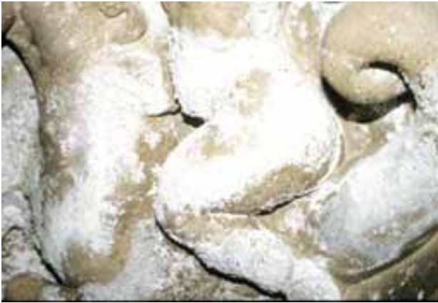
Figure 36. Efflorescence
