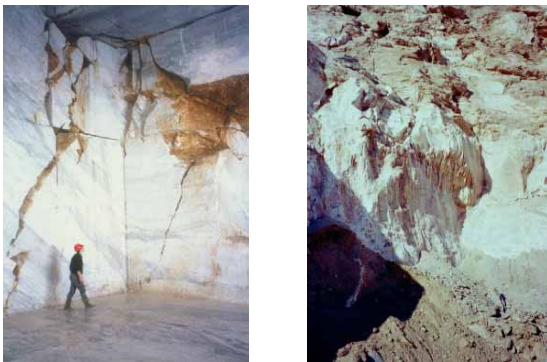
Figure 28. Effects of weathering on a marble. Left: underground mining situation in Carrara (Italy) with small karst caves and strongly weathered discontinuities. Right: open pit marble mine situation near Pentelikon (Greece) with strongly weathered marble layers.
