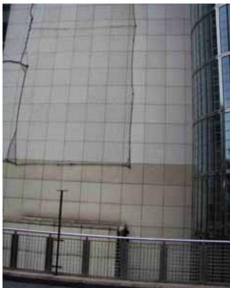
Figure 139. Permanent surface coating. Clearly visible and changing the appearance radically
