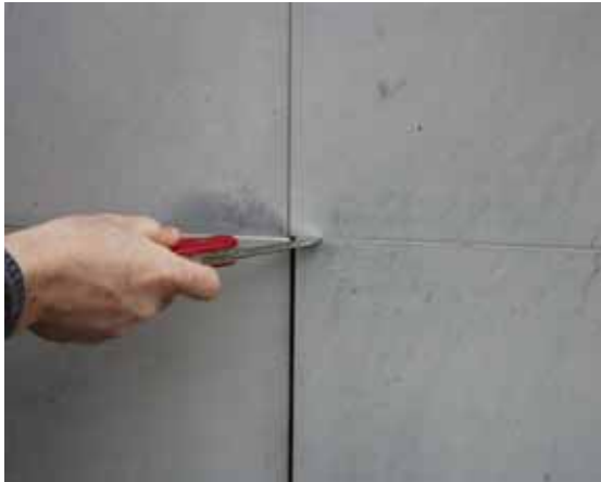
Figure 141. Thermal and hygric expansion may close the dilatation joints and cause cracking
