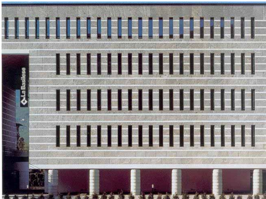
Figure 49. External cladding made of rows of slabs of Indian granite divided by strips of white Carrara marble.
