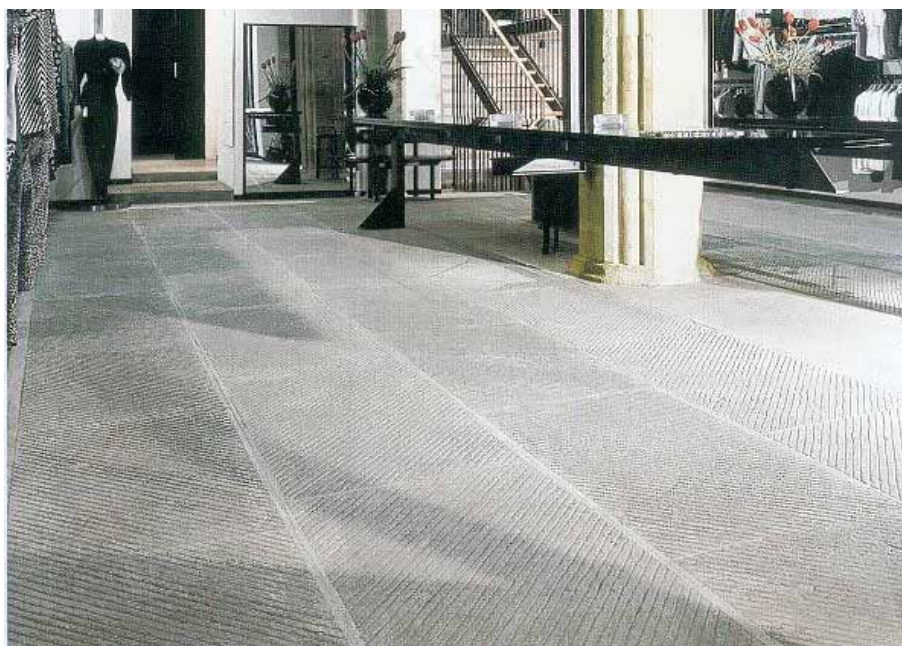
Figure 48. Internal paving of a show room made of slabs of Pietra Serena sandstone.
