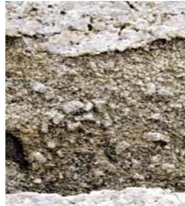
Figure 37. Disaggregation
