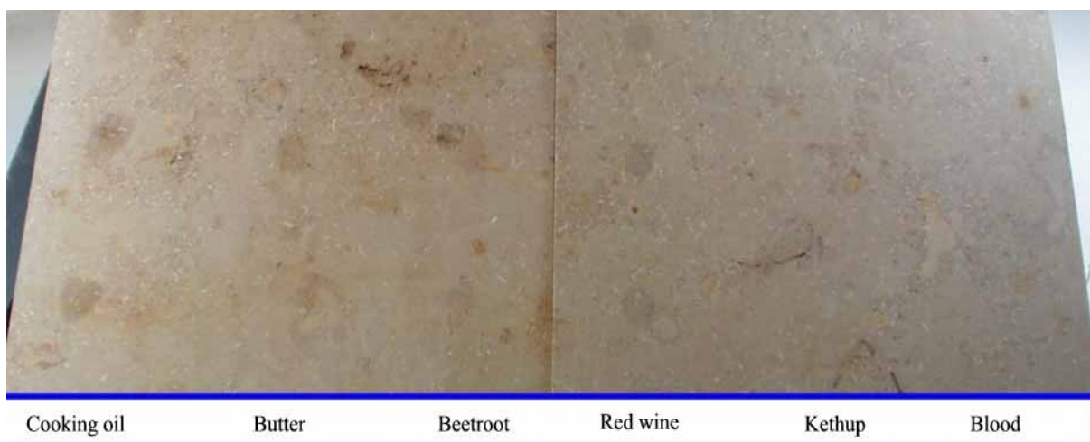
Figure 133. Picture of soap treated limestone after cleaning
