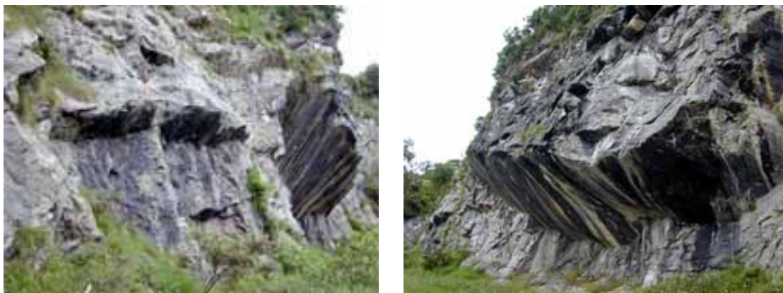
Figure 22. Well defined joint sets controlling the stability/instability conditions in this slope.
