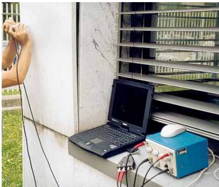
Figure 74. Measurement of pulse velocity on a slab of a marble cladding by surface transmission.
