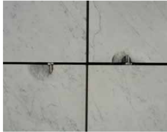
Figure 141. Thermal and hygric expansion may close the dilatation joints and cause cracking
