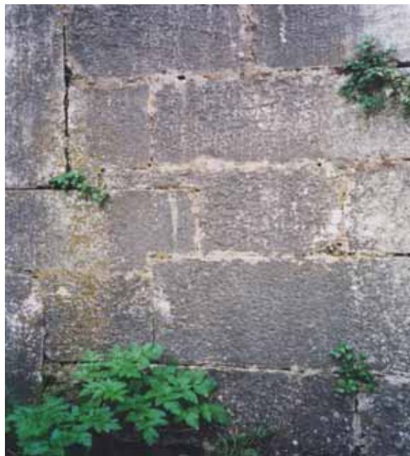
Figure 147. A fortress in Lisbon with biological growth (lichens on surface and weeds in joints)
