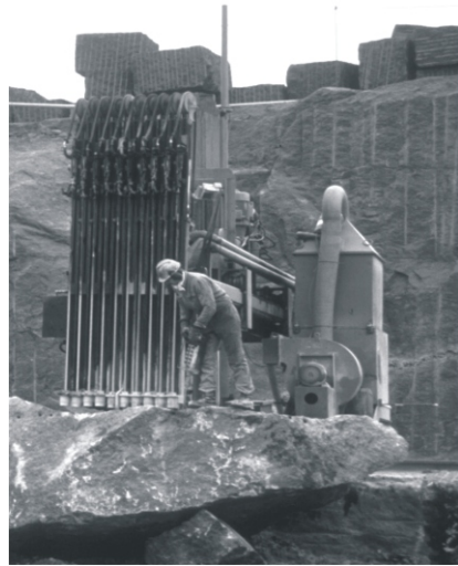
Figure 20. Multi-hammer, hydraulic drill for squaring of blocks.
