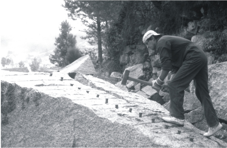
Figure 24. Worker using short plugs for wedging granite block in Vigo, Spain.
