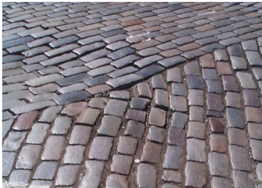
Figure 23. Rotation of setts as a result of traction forces
