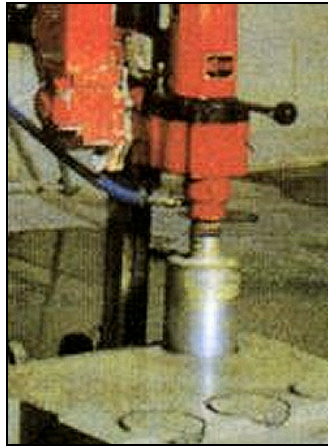
Figure 155. Drilling machine in operation
